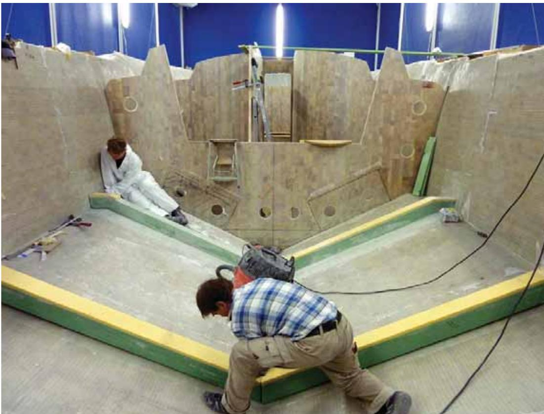
A mixture of WEST SYSTEM resin/hardener and 403 Microfibres should be spread into the open cuts: the panel is then bent over a temporary jig of its final shape and temporarily clamped until the epoxy cures. Fill the internal angle, with a 20mm radius of modified epoxy and allow to cure. Apply an additional layer of fibreglass cloth to the inside of the angle, overlapping the fillet by 25mm on each side.
